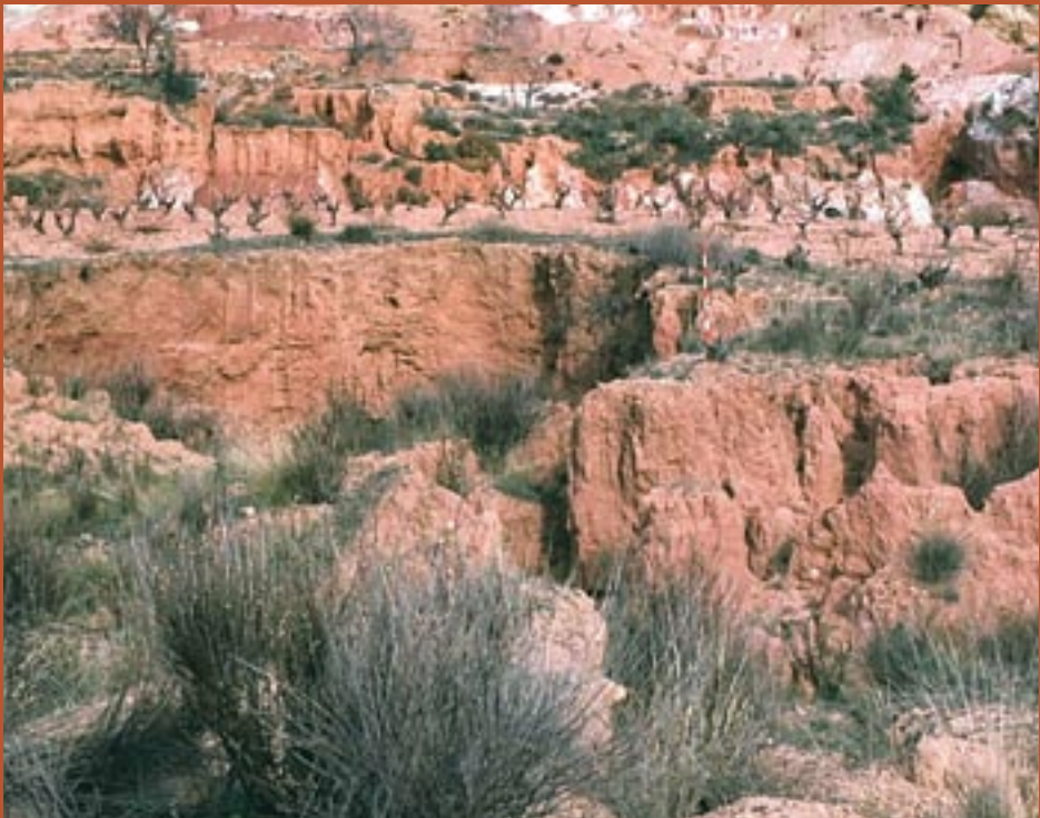
Collapse of abandoned agricultural (almond tree and vineyard) terraces near Valencia, Spain.
