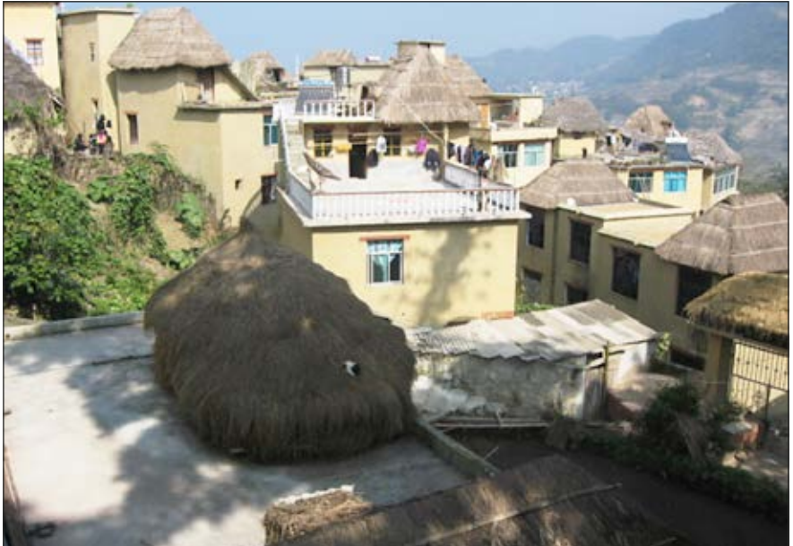
Plate 1: The distinctive 'mushroom houses' of the Hani minority in Qingkou village, Yuanyang. Rice straw provides the 'thatch' (roofing materials). Photo taken by Mike Fullen (Wolverhampton, UK) on 12 November 2010.
