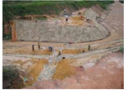
Partial view of the protected soil surface, with Buriti geotextiles.
