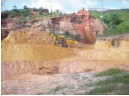
The beginning of the rehabilitation work.
