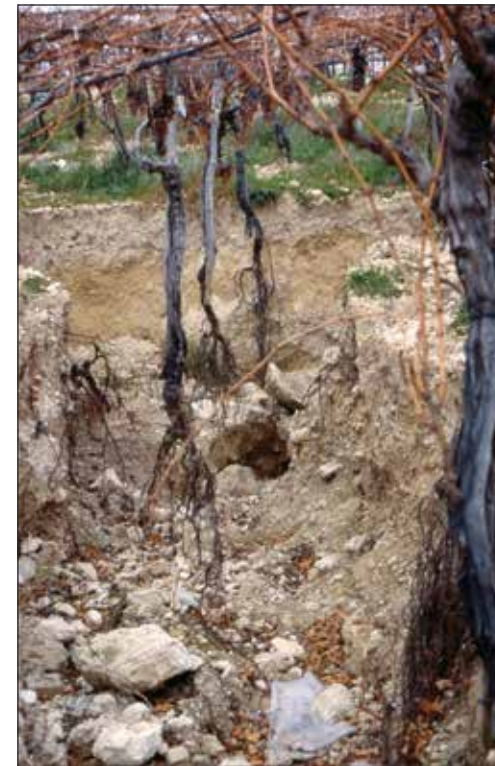
Plate 2: Deep gully erosion in anthropogenic soils under vineyards in the Canicatti area of central Sicily, Italy (photo by C. Dazzi).
