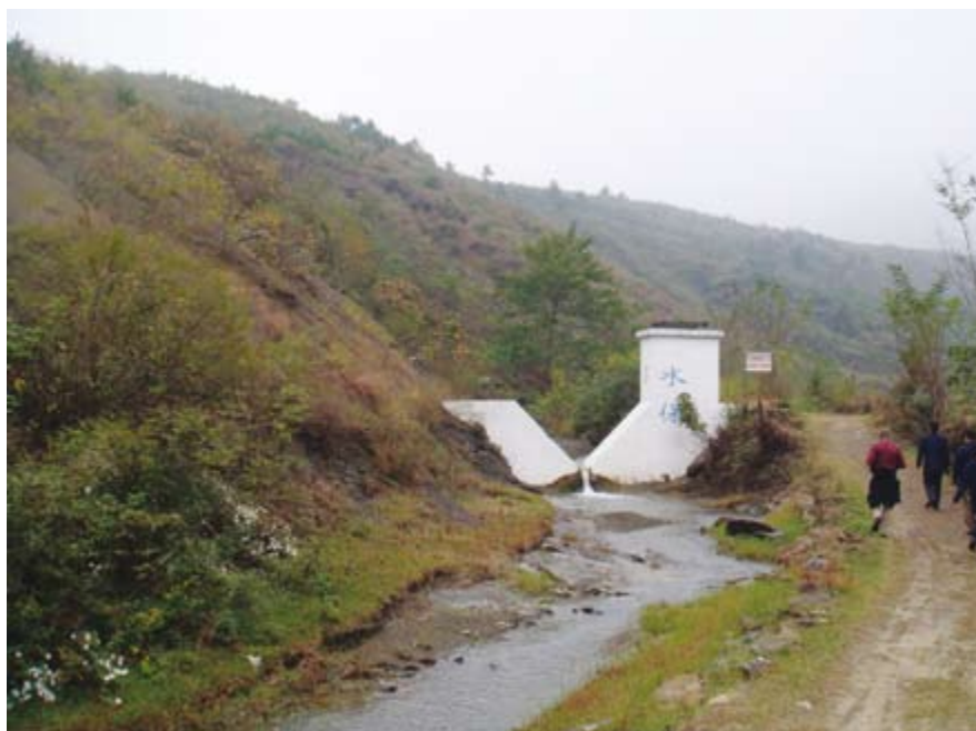
Soil conservation project in Yiling, Hubei Province, China (October 2008). Soil erosion occurred as a result of deforestation. An afforestation programme was implemented to decrease sediment reaching the river channel.
