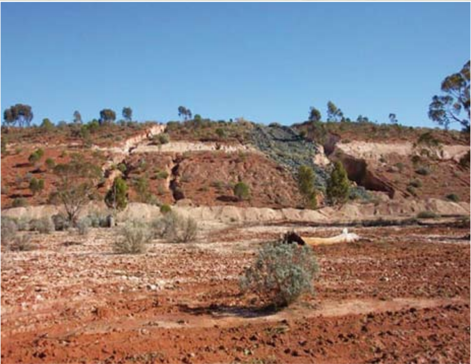
Cover photo: Examples of gully erosion through berms on waste dumps in the arid Goldfields region of Western Australia (photo from Rob Loch, Harlaxton, Queensland, Australia).
