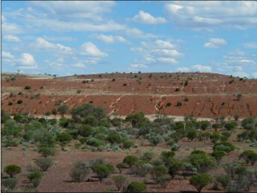
Plate 5. Examples of gullying through berms on waste dumps in the arid zone (~220 mm/y rainfall).
